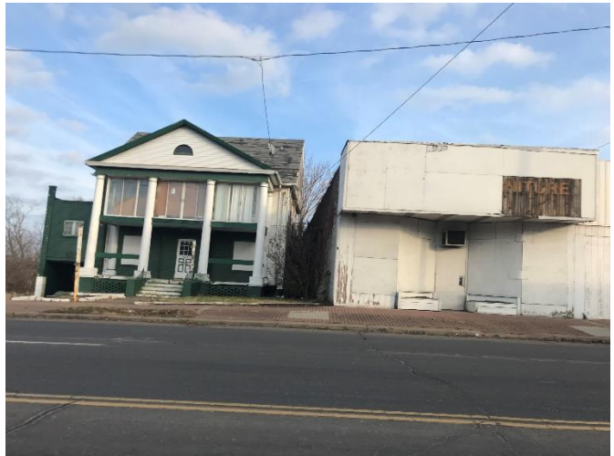
2. Vacant commercial buildings
