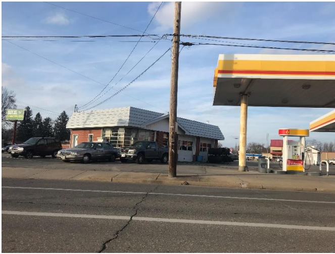
1. Shell gas station
