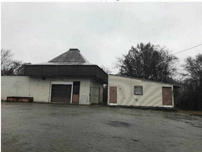
5. Vacant commercial building
