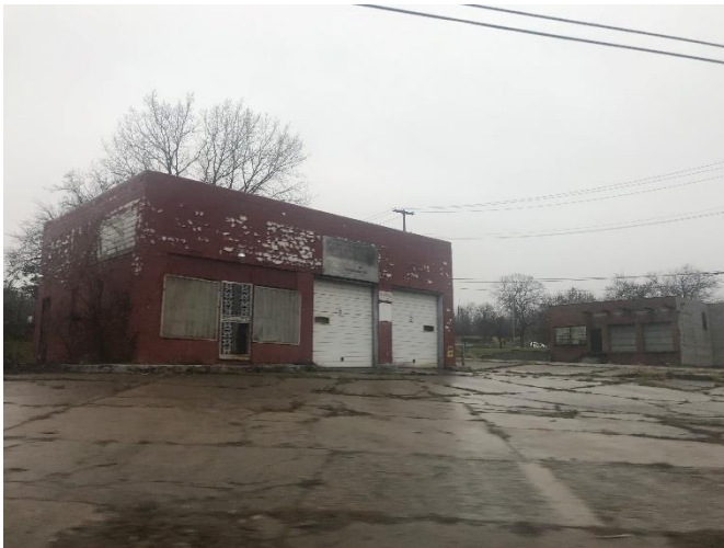
3. Vacant commercial building
