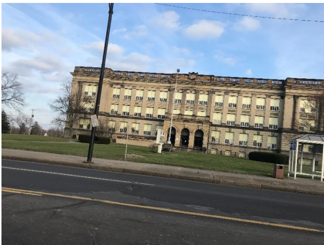
5. Vacant school building
