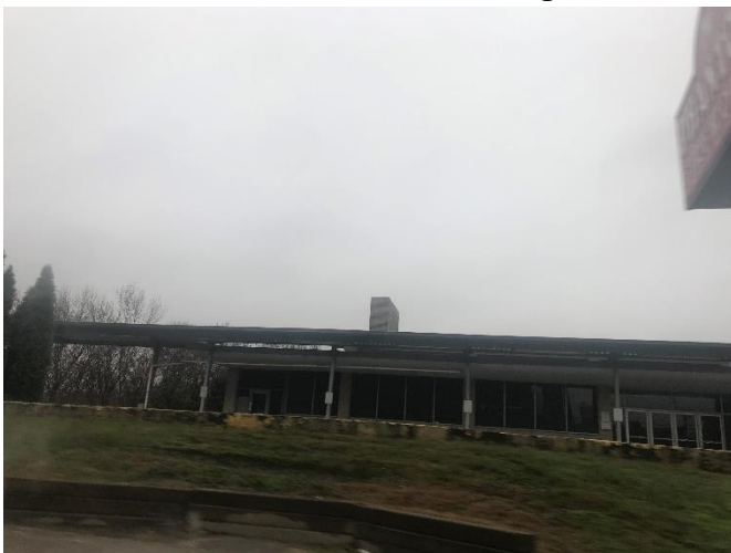
5. Vacant commercial building
